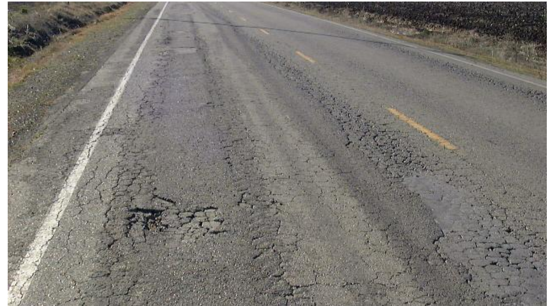
Extensive and likely deep alligator cracking, Starting to form potholes
